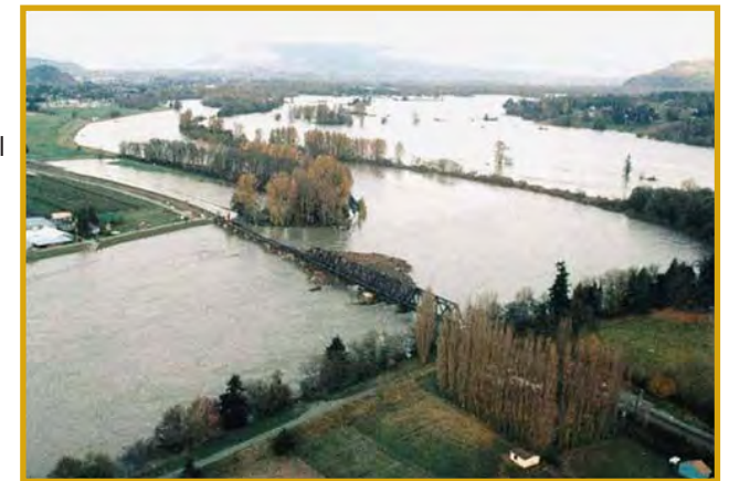
BNSF Skagit River Bridge during Flooding
