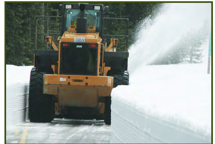
Roadway Maintenance on State Route 20
