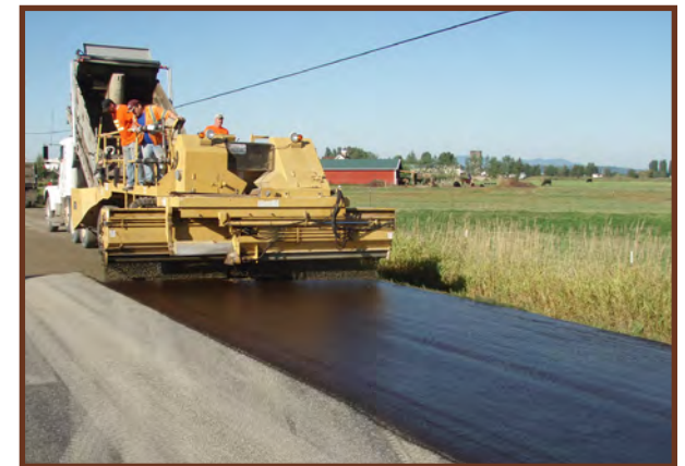
Roadway Resurfacing in Skagit County
