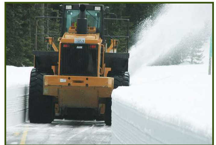
Roadway Maintenance on State Route 20
