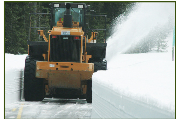
Roadway Maintenance on State Route 20
