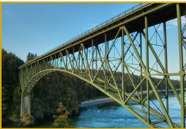
Deception Pass Bridge to Island County
