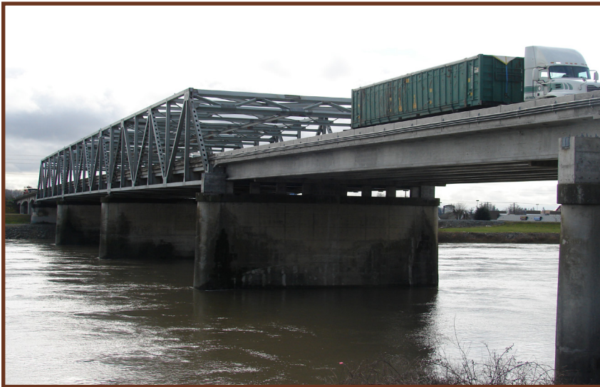
Interstate 5 Bridge over Skagit
