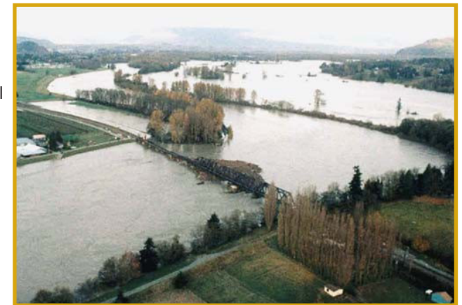
BNSF Skagit River Bridge during Flooding
