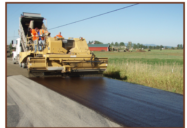
Roadway Resurfacing in Skagit County
