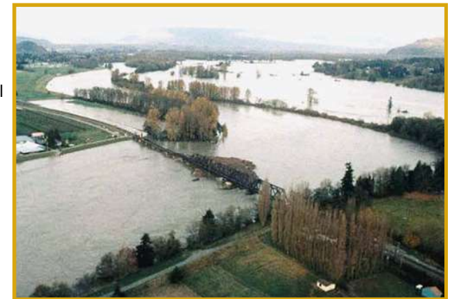
BNSF Skagit River Bridge during Flooding
